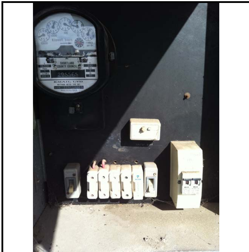
Photo 56: 16 Bowditch Avenue – Zelemite backing board to the power box of the house
