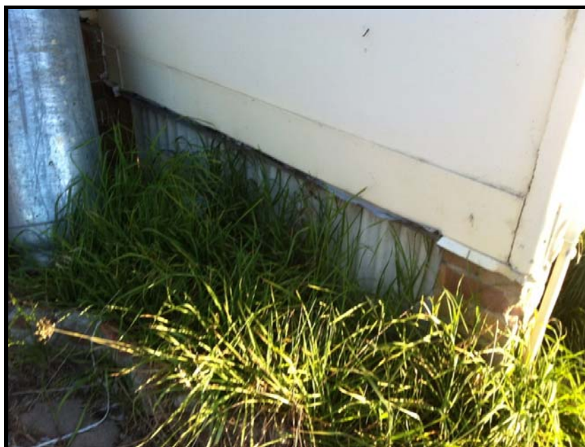
Photo 22: 8 Bowditch Avenue - section of corrugated AC sheeting used as infill panel near the steps to the side entry to the house.
