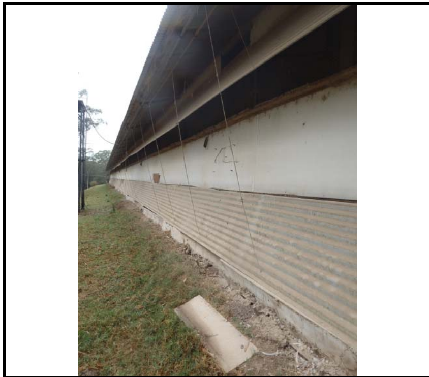
Photo 4: 18 Bowditch Avenue - Example of ACM sheeting on exterior wall lining to the northern chicken shed
