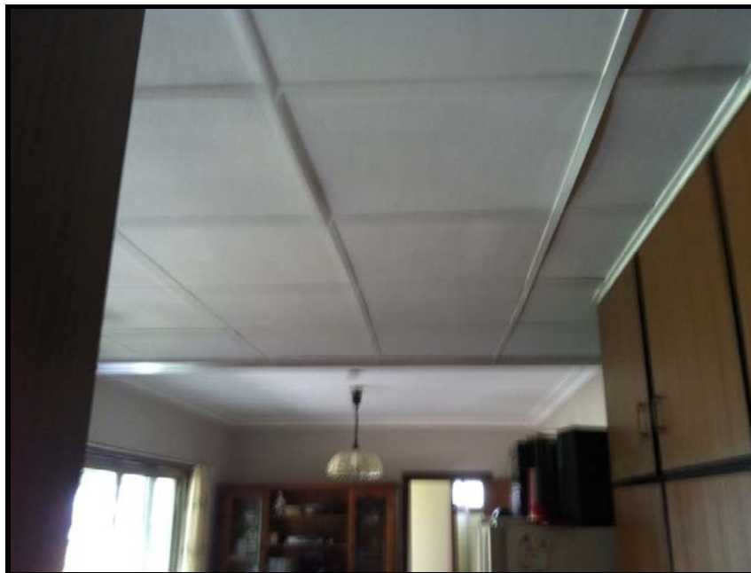
Photo 39: 14 Bowditch Avenue – ACM square panels use in false ceiling above the kitchen in the house.
