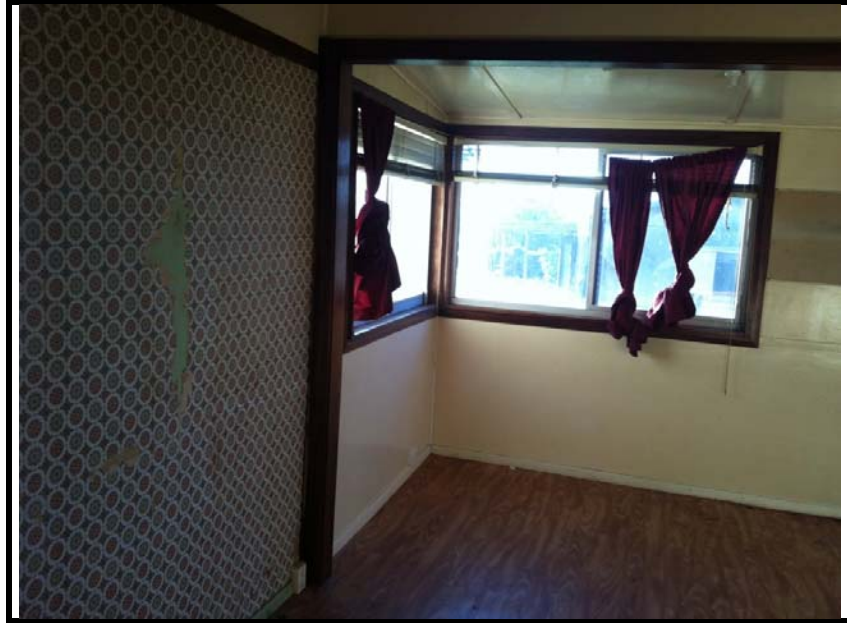
Photo 19: 8 Bowditch Avenue - AC sheeting lining the walls and ceiling to the back room of the house.
