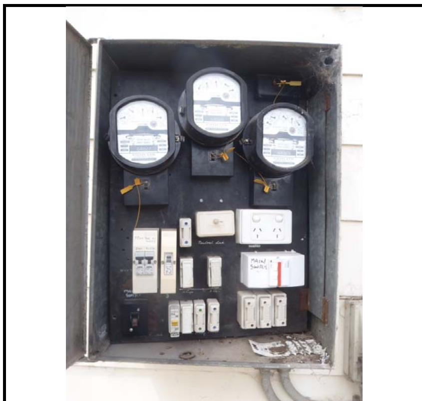
Photo 5: 18 Bowditch Avenue – zelemite electrical backing board
