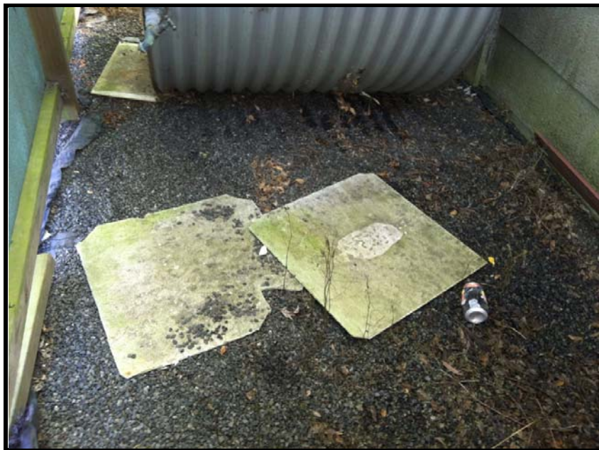
Photo 45: 14 Bowditch Avenue – ACM square panels (appear to be as use in false ceiling above the kitchen in the house) on the ground in the shed at rear of the house.
