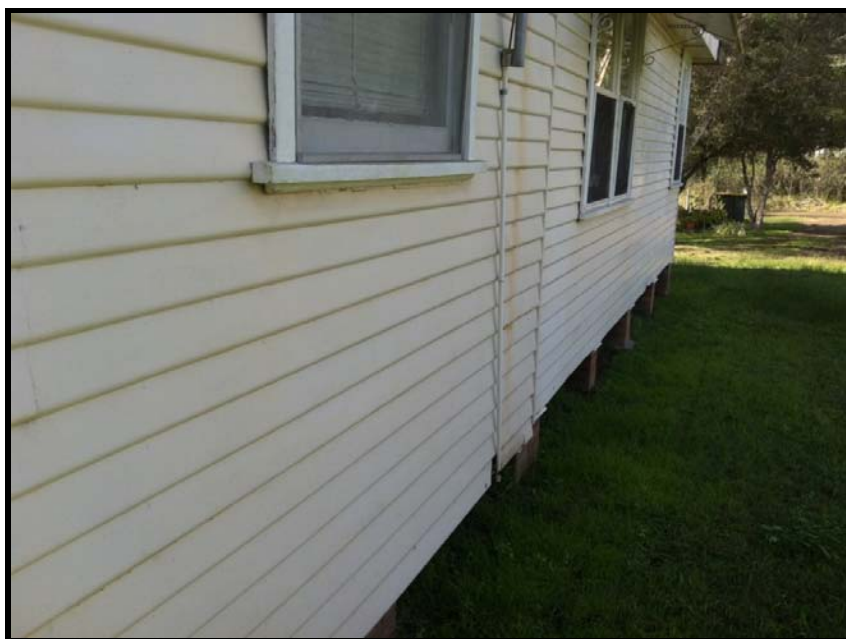
Photo 54: 16 Bowditch Avenue – Corrugated ACM sheeting of “weatherboard” appearance to the exterior walls of the house.
