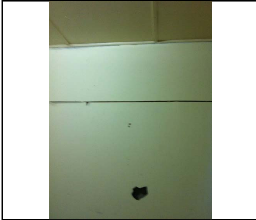
Photo 13: 8 Bowditch Avenue - section of AC sheeting lining to wall and ceiling to bedroom adjacent to the front (western) room of the house
