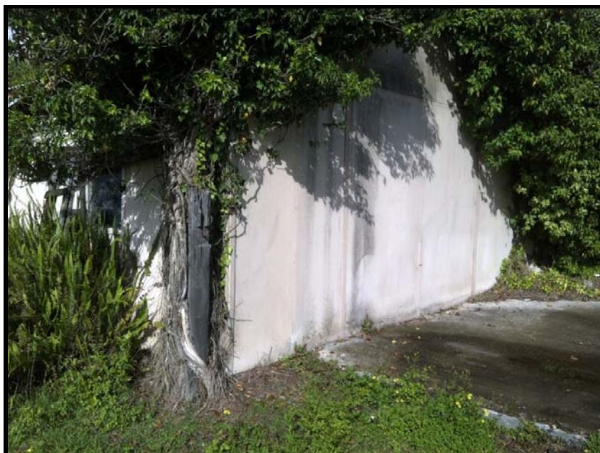
Photo 58: 16 Bowditch Avenue – ACM sheeting used to the sides and rear walls of the shed/ garage.
