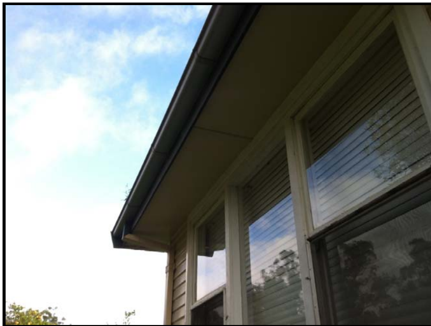
Photo 53: 16 Bowditch Avenue – Section of the ACM sheeting used to eaves to all sides of the house
