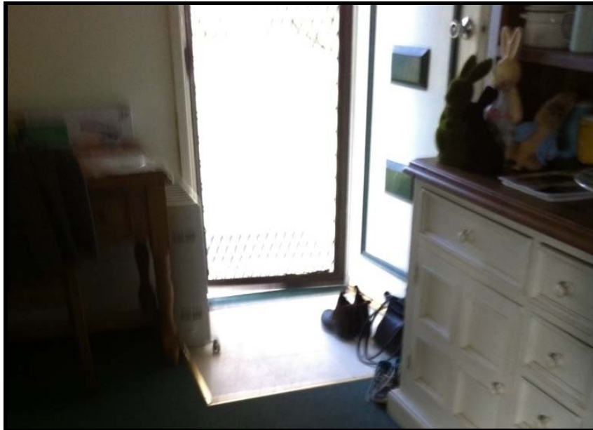
Photo 52: 16 Bowditch Avenue – Vinyl floor tiles that are potentially ACM (undamaged and due to location in inhabited house no sample taken) at the front door of the house
