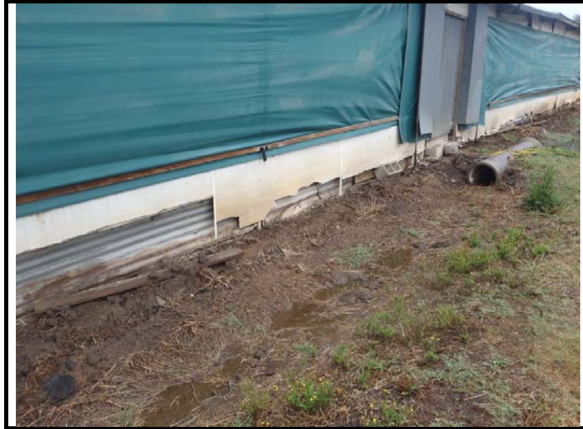
Photo 1: 18 Bowditch Avenue - Example of ACM sheeting on exterior wall lining to the southern chicken shed
