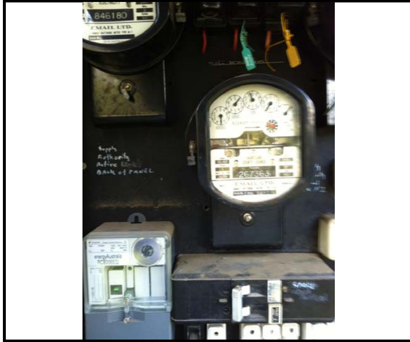
Photo 29: 12 Bowditch Avenue – Zelemite backing board to the older power box on the house
