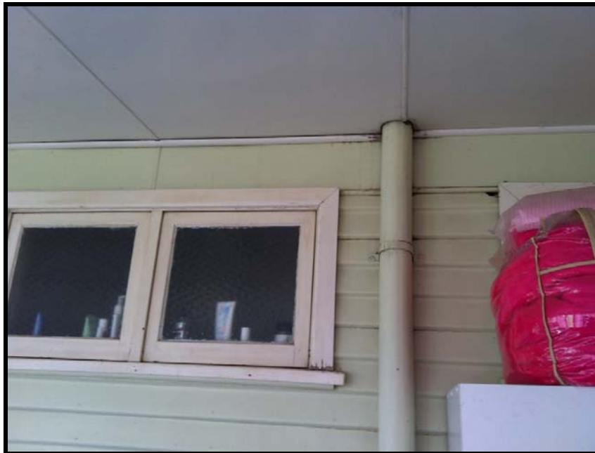
Photo 50: 16 Bowditch Avenue – ACM flat sheeting lining wall (panel above weatherboards) and ceiling of enclosed back verandah of the house. Also showing corrugated ACM sheeting of “weatherboard” appearance.
