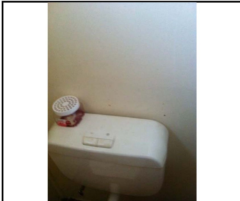
Photo 30: 12 Bowditch Avenue – ACM sheeting lining the walls to the toilet room in the rear of the house
