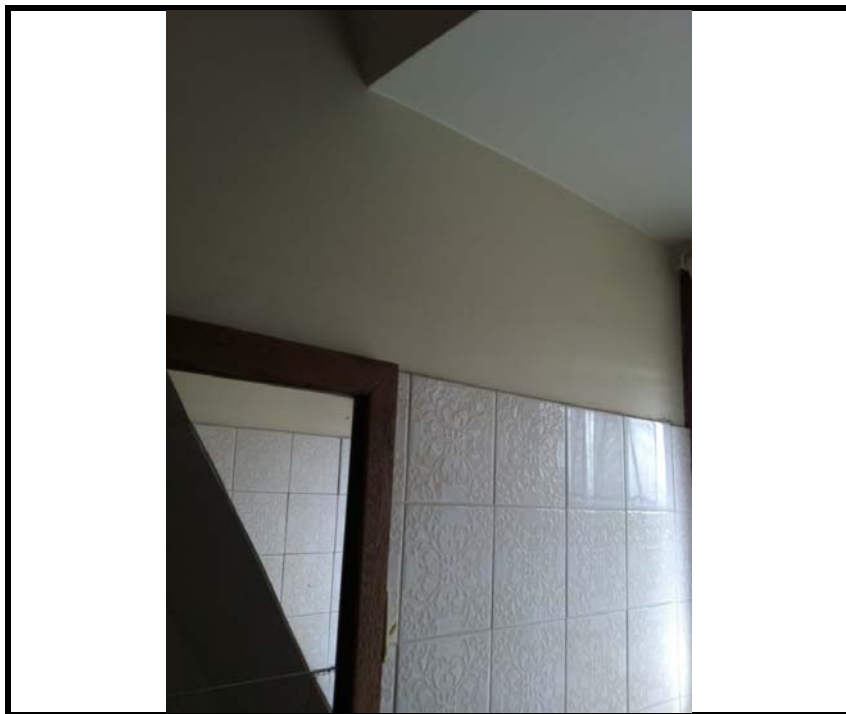
Photo 41: 14 Bowditch Avenue – Painted and tiled ACM sheeting lining the walls in the first floor bathroom of the house
