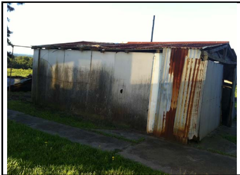
Photo 23: 8 Bowditch Avenue - Section of the AC sheeting lining the walls to the garage.
