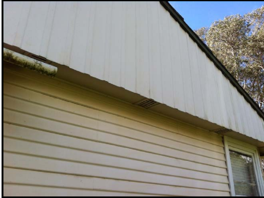
Photo 55: 16 Bowditch Avenue – Corrugated ACM sheeting to the gable ends of the house.
