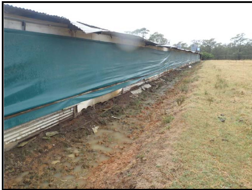
Photo 2: 18 Bowditch Avenue - Example of ACM sheeting on exterior wall lining to the southern chicken shed. Note varying sized fragments in the adjacent soils
