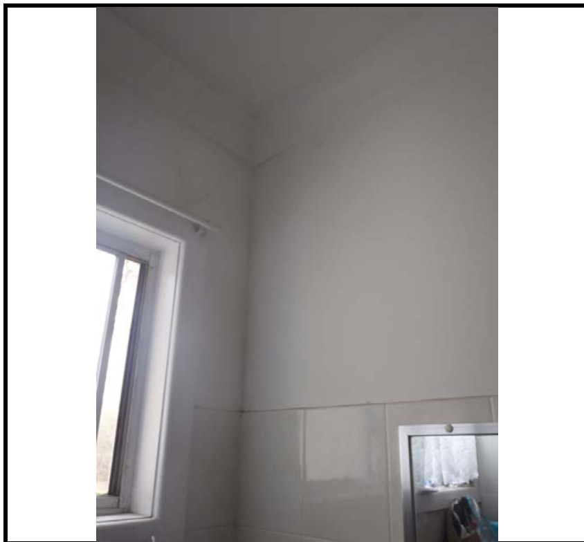
Photo 9: 18 Bowditch Avenue - example of ACM sheeting walls in bathroom
