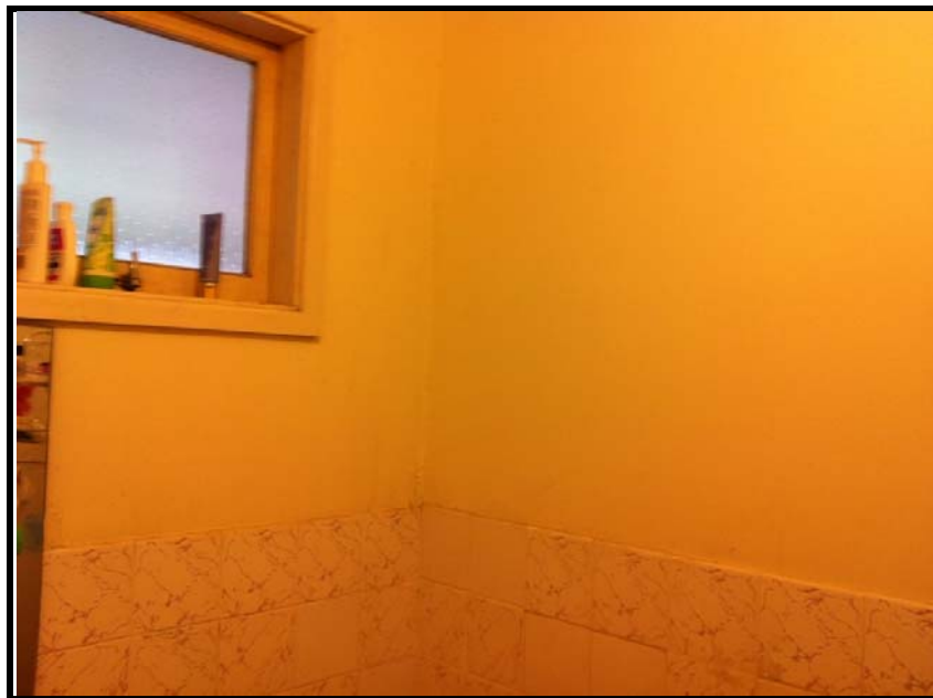
Photo 47: 16 Bowditch Avenue – ACM sheeting lining the walls of the bathroom in the house
