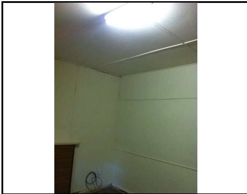
Photo 14: 8 Bowditch Avenue - AC sheeting lining the walls and ceiling to the front (eastern) room of the house
