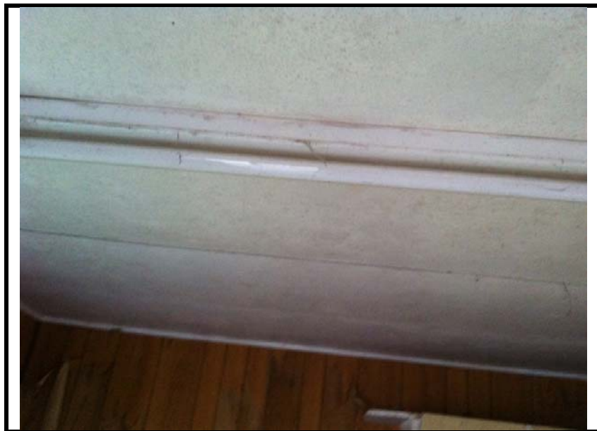
Photo 25: 8 Bowditch Avenue - fluorescent light and AC sheeting lining the ceiling in the front (south) room of the shed.
