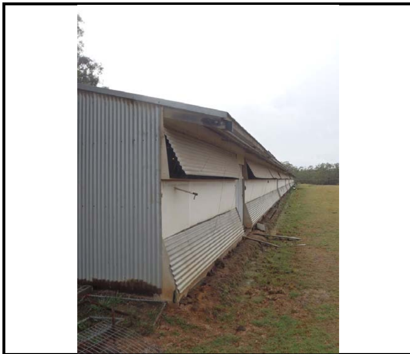
Photo 3: 18 Bowditch Avenue - Example of ACM sheeting on exterior wall lining to the northern chicken shed
