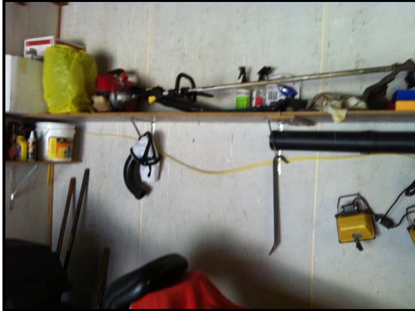
Photo 35: 14 Bowditch Avenue – ACM sheeting lining to rear wall of garage to house
