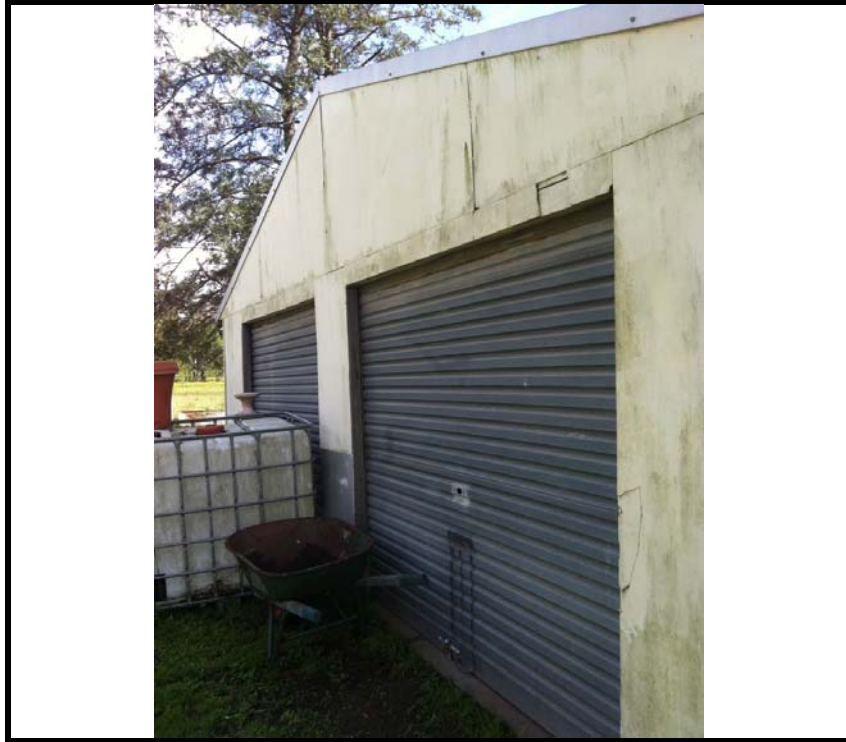
Photo 33: 12 Bowditch Avenue – A section of the ACM sheeting lining the exterior of the garage
