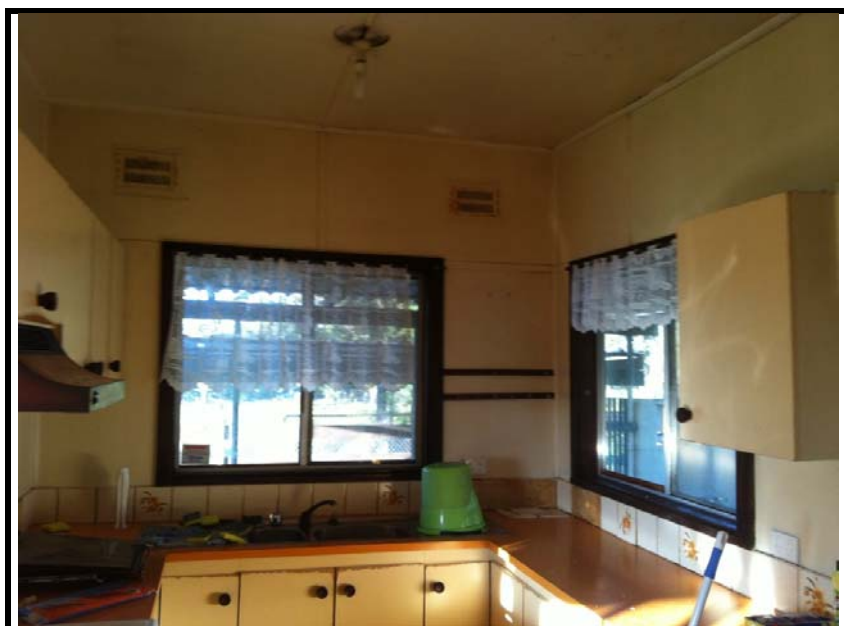
Photo 18: 8 Bowditch Avenue - AC sheeting lining the walls and ceiling to the kitchen of the house.
